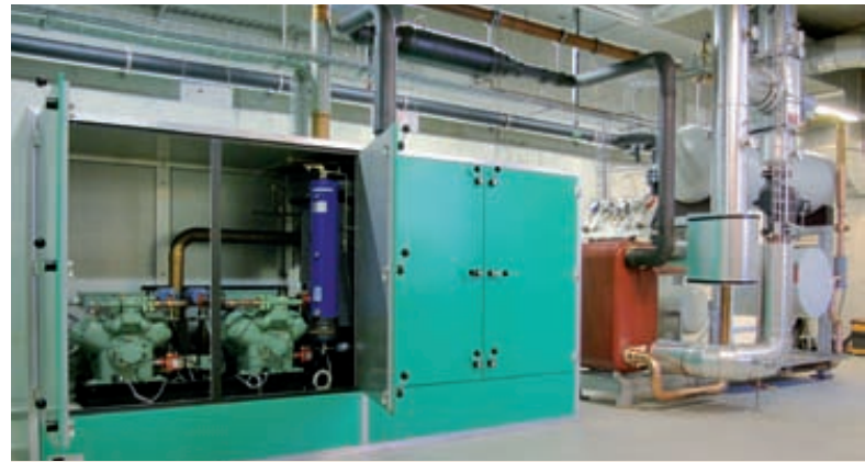
Heat pumps serving multiple functions are particularly advantageous. Research and development are concentrated in this area in order to further improve the efficiency and integration of systems in the technical building services. In this picture, a 450 kW heat pump draws its power from a gas-engine-powered combined heat and power generation unit. It is an element in the energy system of a large building complex.
