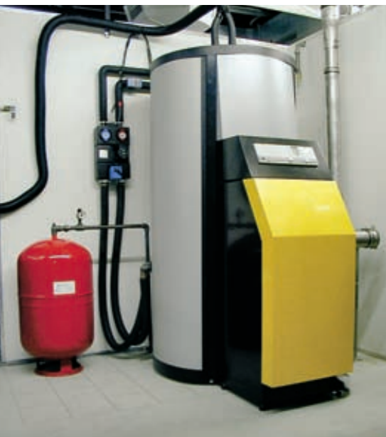
Compact combi-systems for domestic water heating and space heating are tested at the University of Applied Sciences in Rapperswil. Promising results indicate that a significant improvement in solar heat delivery at less cost may be achieved, thanks to compact design and system optimisation.
