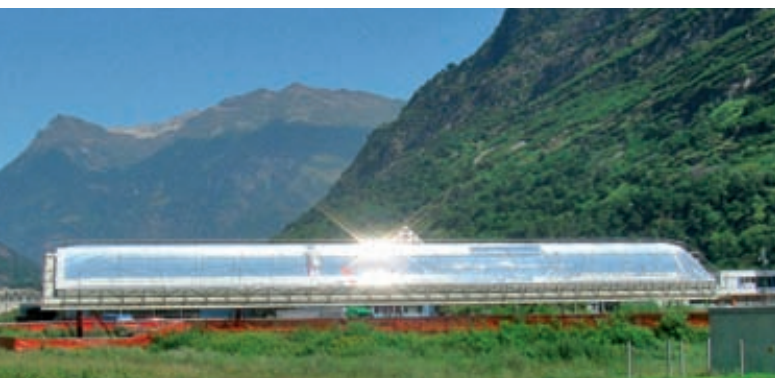
The third prototype put into operation at the site of AirLight Energy in Biasca. The concentrating collector has a linear construction and it makes use of the very simple, new concept of flexible, pneumatic reflectors. The membrane is attached to a simple frame of prefabricated pre-stressed concrete.
